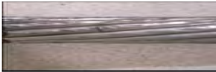
Figure 31 shows example of fretting conductor fatigue failure risk in AA or ACSR conductor
