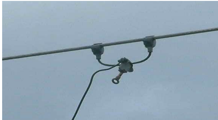
Figure 10: Live line clamp connected via D-clamp
