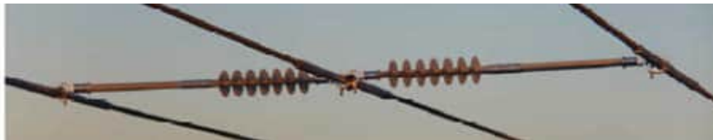
Figure 21 shows a HV mid span spacer set for AAC damping galloping solution
