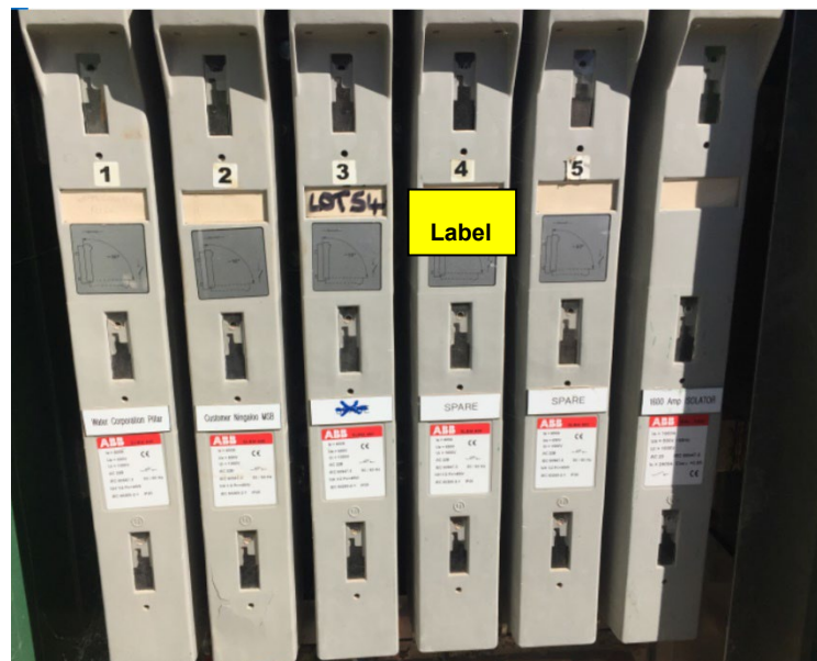
Figure 28 – ‘ABB’ Fuse Switch label location.
