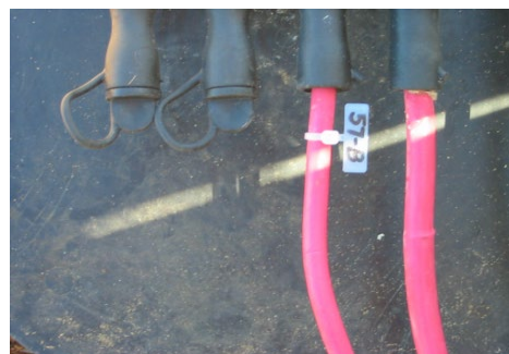
Figure 40 – Consumer Service Cable ID Tag label examples.
