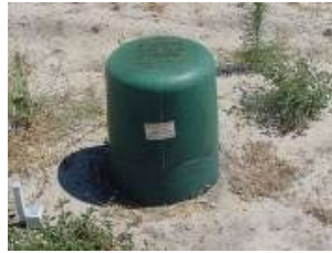
Figure 31 – Universal Pillar with Normally-Open point marked with ‘I’.
